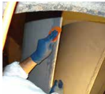
Forming and rebuilding
