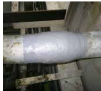
Wrapping and patching
